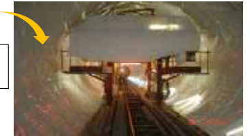
Application of waterproof sheet in tunnel
