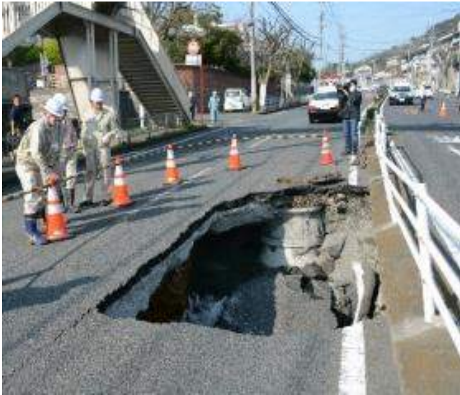
Fig.1 Road collapse accident due to sulfuric acid degradation of sewer pipe
