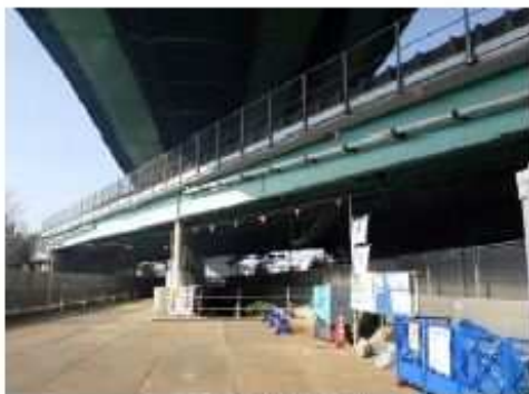
吊り足場架設前
